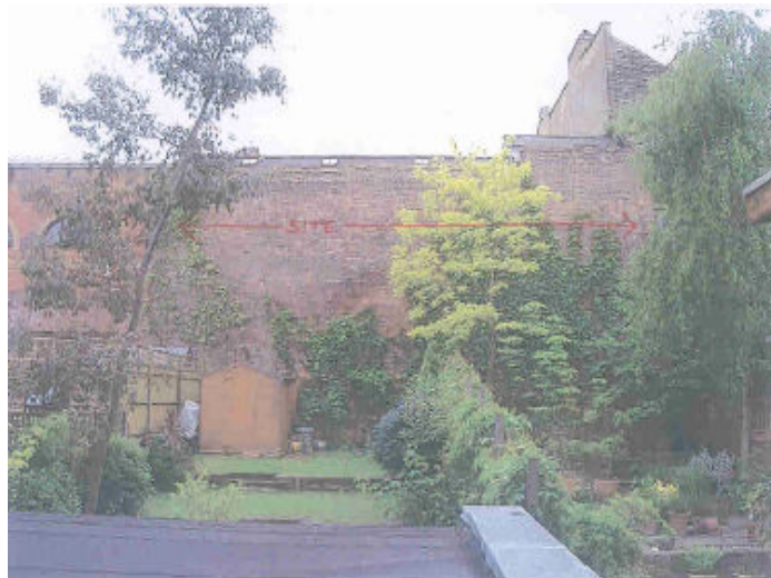
Views from Holmesdale Road
