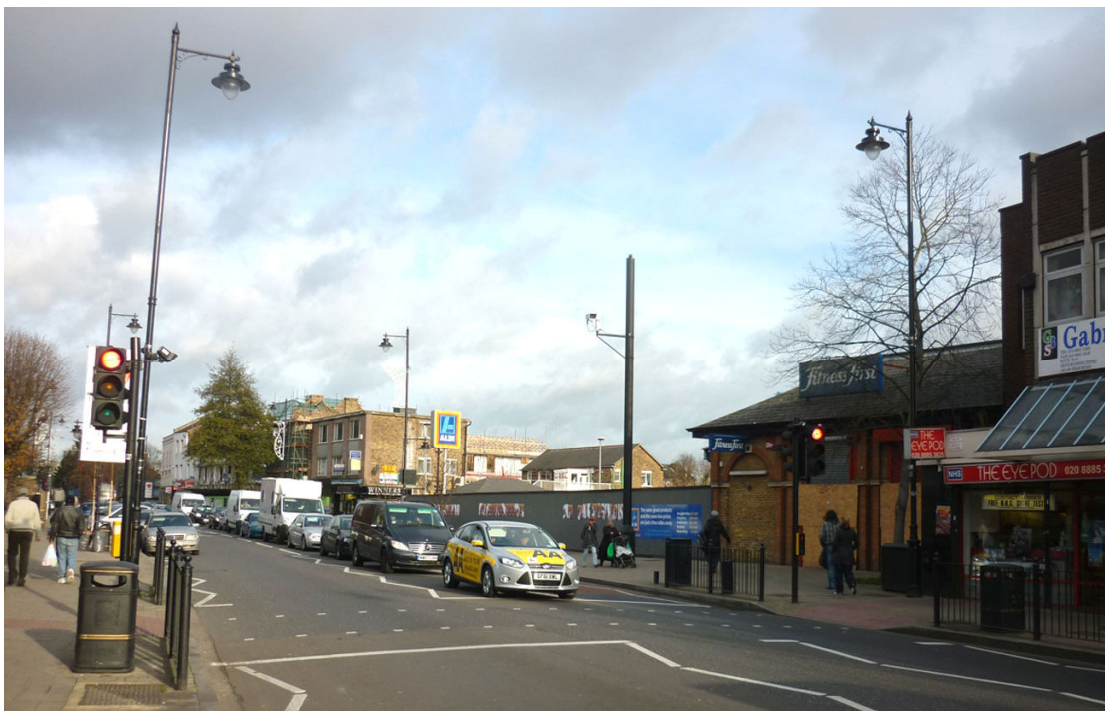
View of the site from High Road post demolition
